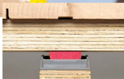
J-Lock component in unloaded position.
